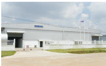
THAILAND THAI KYOWA GMB CO., LTD. 304 Industrial Park, 410/1 Moo 7 Tambol Tha Toom, Amphur Srimahaphote Prachinburi 25141, Thailand
