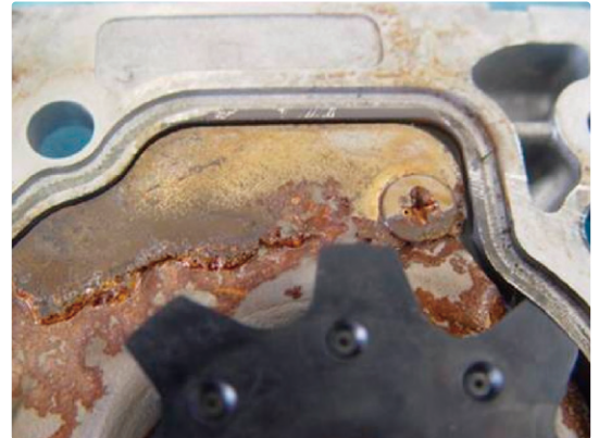
Bottom plate corrosion
